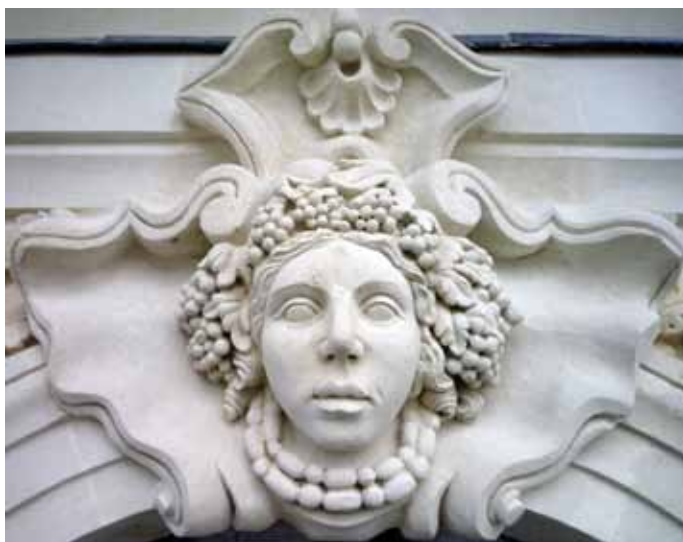
'FLORE', 35" X 24", TUFA STONE. CARVED TO REPLACE AN OLD ONE IN NANTES, FRANCE
