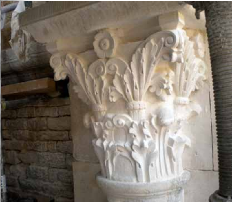
A REPLACEMENT CHAPITEAU, 24" X 36", FRENCH LIMESTONE. CARVED IN THE ROMAN ART TRADITION FOR THE ABBAYE DE CLUNY IN BURGUNDY FRANCE.
