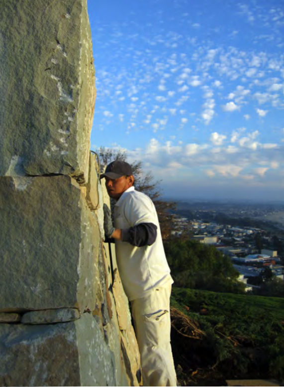
SUMINORI CHECKING BATTER AND CURVE OF THE WALL, OBLIVIOUS TO MY TAKING HIS PICTURE
